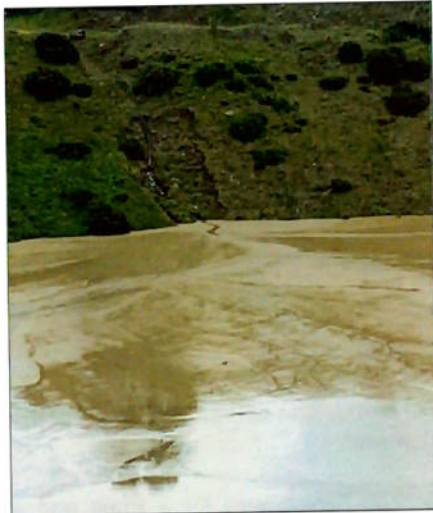
Silted pond within the substitute consent application boundary
