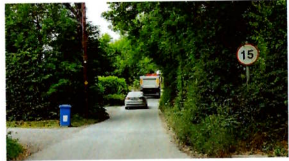
Quarry traffic using inadequate lane
