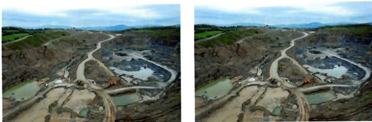
Figure 4.1 Drone Footage April 2023 (LHS) and May 2023 (RHS)
